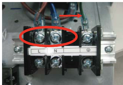
< Input Power Source Check Point >
